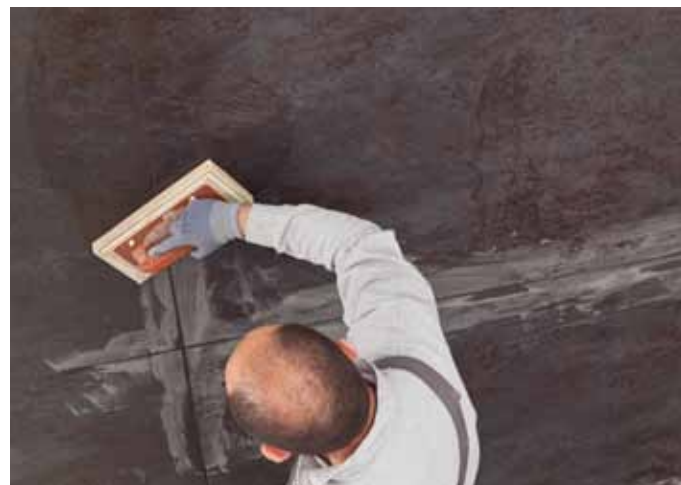
fig.39 / Stuccatura. / Grouting.
